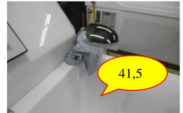
If the temperature is set at 42 ° C (anti-scalding), the corresponding display "HOT" alternates with the temperature and the water flow is switched off.
