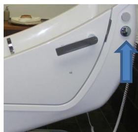
Open the screw connection by turning it counterclockwise
